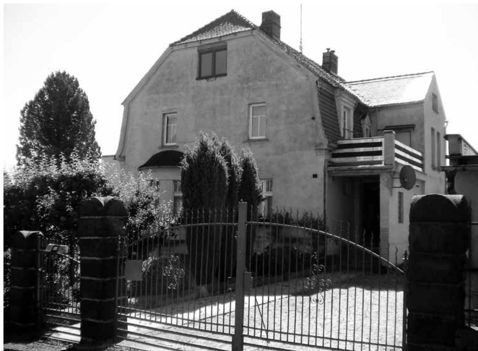
House on today's November 17 th Street in Šluknov, where Kuncewicz's group was staying on 6 July 1945 (state in 2015; photo: J. Friedl)
